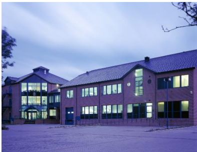
Figure 1: Headquarters of Plextek Consulting, Great Chesterford, United Kingdom.
