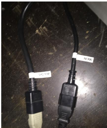
From the rear bottom of the equipment rack extend two power inlet cables, one for the PXI chassis and one for the rest of the system. These cables are IEC C14 types and can be easily customised with location specific IEC C13 power cords.
