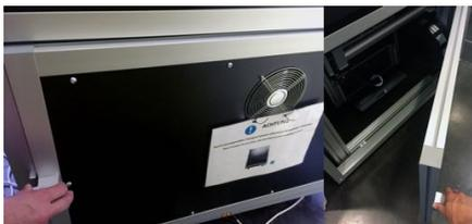
The equipment rack has a door on the rear and front side for easy access to the rack equipment and wiring. Open the door by lifting the handle as indicated on the picture on the left.
