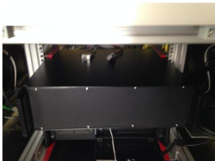
When the wiring is complete slot the IEICE<sub>y</sub> in the centre mounting rail of the rack as shown.
